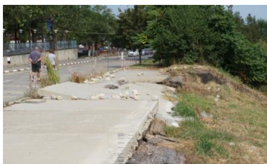
Fig. 3.5. c and d. - Landslides under the promenade alley/sidewalk Eforie South
