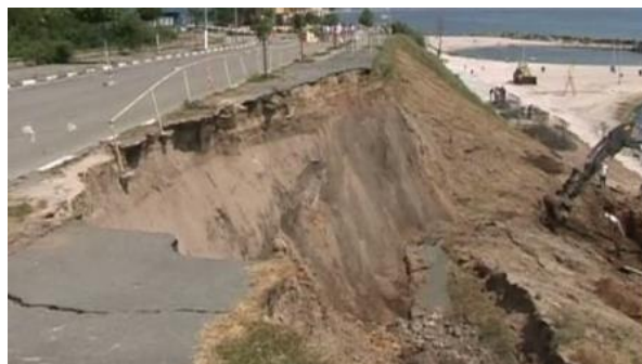
Fig. 3.5. c and d. - Landslides under the promenade alley/sidewalk Eforie South
